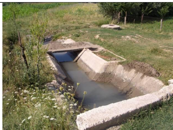
Photo 1: Hydropost discharge measurement structure at the intake to a WUA command area
