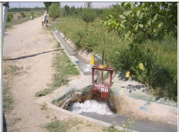
Simple control gate at division point within the WUA command with sharp-crested Cipoletti measuring weir in the channel in the background
