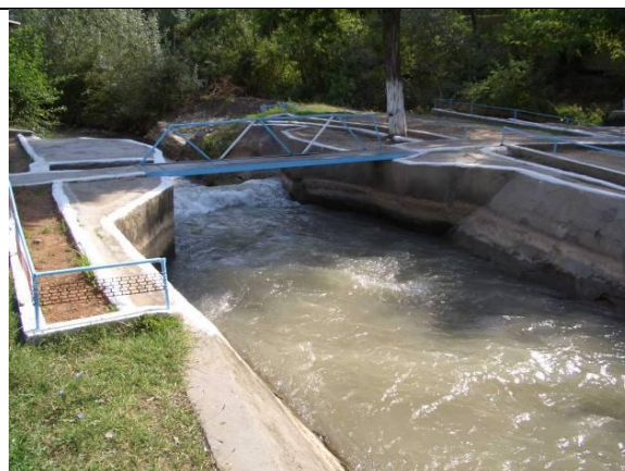
Photo 2: Hydropost discharge measurement structure at the intake Federation of WUAs command area
