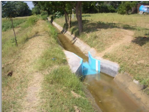
Cut-throat flume measuring device within a WUA command area on the Dharoi Irrigation Scheme.
